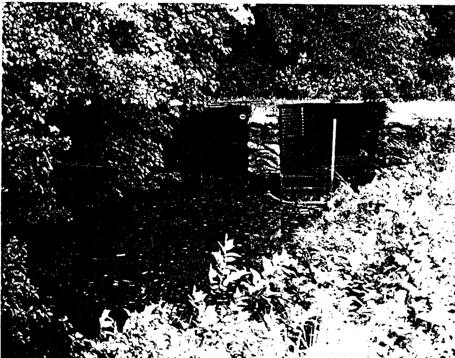
Below: Watershed-scale, flash-board riser-type water control structure(s) installed in main channel in Perquimans County, North Carolina. Upstream watershed drainage area controlled by structure is about 2,500 acres. Effective length of the weir, that is, the combined width of the two structures, is 12 feet.
