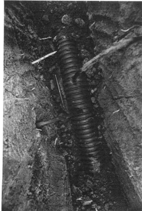
Fig. 3. Barbed fitting at the end of the pipe used for jetting a hole from the trunk of each tree to the trench containing the corrugated pipe. The delivery hose is slipped over this fitting and is thereby drawn into the hole when the jetting pipe is retracted.
