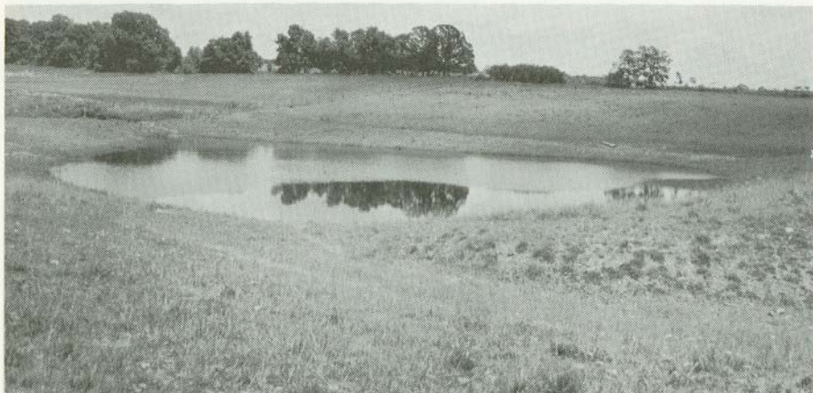
Fig. 11—The Dade County pond one year after treatment. At this time, it was filled to a depth of 7.4 feet—near the upper limit of the blanket-treated part of the basin.
