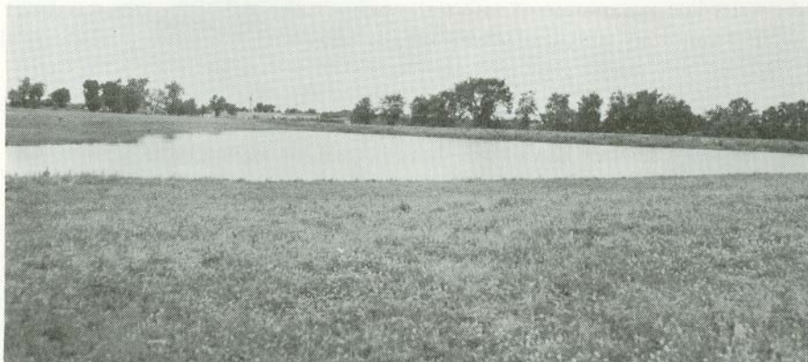
Fig. 7—This pond in Greene County leaked badly. Since treatment above the water line with hexametaphosphate and a silt loam blanket, the pond has remained filled to the treated level. Water that collects above this level during heavy runoff seeps away rapidly.
