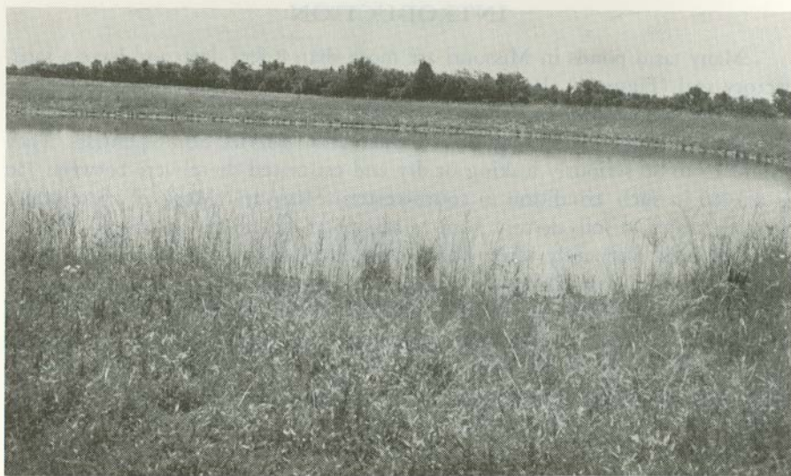
Fig. 3— A shallow pond that has no seepage problem. Because of reduced storage volume, shallow ponds may go dry due to evaporation during sustained periods of drouth. It may be necessary to increase the storage volume by increasing the area of the excavation and height of the dam, rather than cutting deeply into permeable cherty layers.
