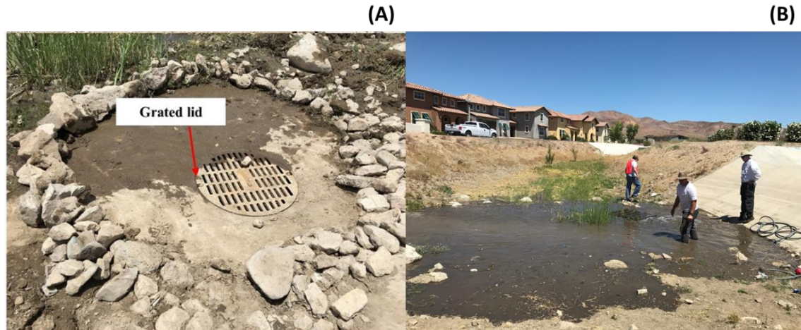
Figure 1. The DW1 (A) and the falling head test was conducted by flooding the basin using a fire hydrant and filling and draining DW1 on June 5, 2017 (Sasidharan et al., 2018) (B), by UC Riverside and USDA Riverside.
