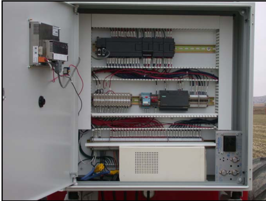
Figure 5. Photograph of the interior of the wiring cabinet showing the PLC, power supplies, wiring and front interface panel.
