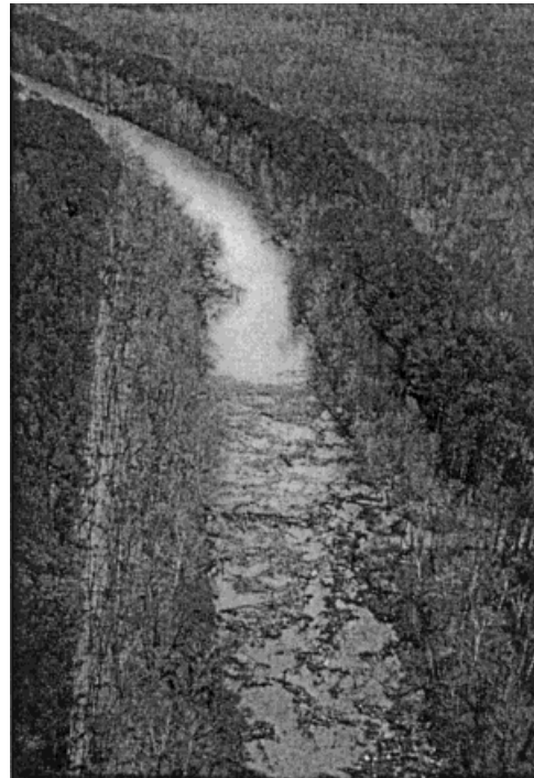
Figure 4. Upstream end of sediment and debris blockage in Yalobusha River, 1997
