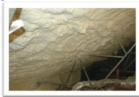
Spray-on expanding foam insulation on the attic ceiling
