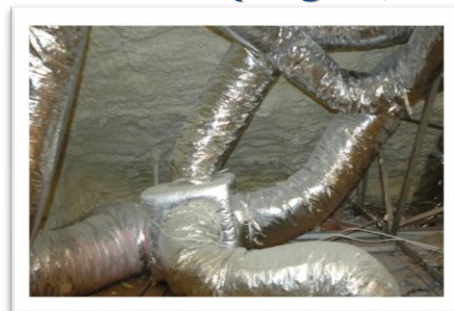
Insulation of ductwork and pipes
