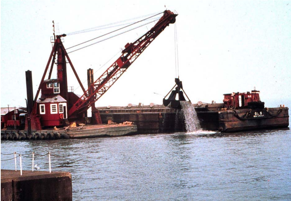
Figure I-2: More dredging of Toledo Harbor
