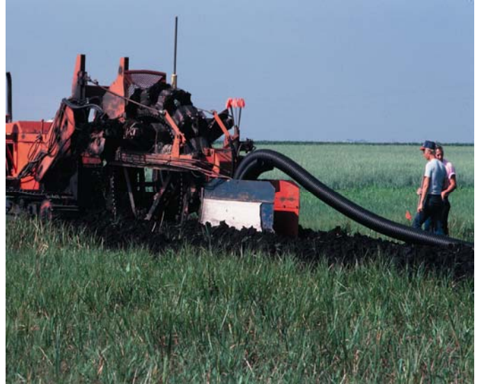
Figure VI-3: Tile drainage was shown to reduce erosion and sediment load from the watershed.
