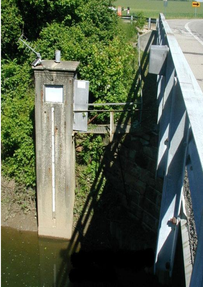
Figure II-4: USGS stream gage downstream from Fort Jennings
