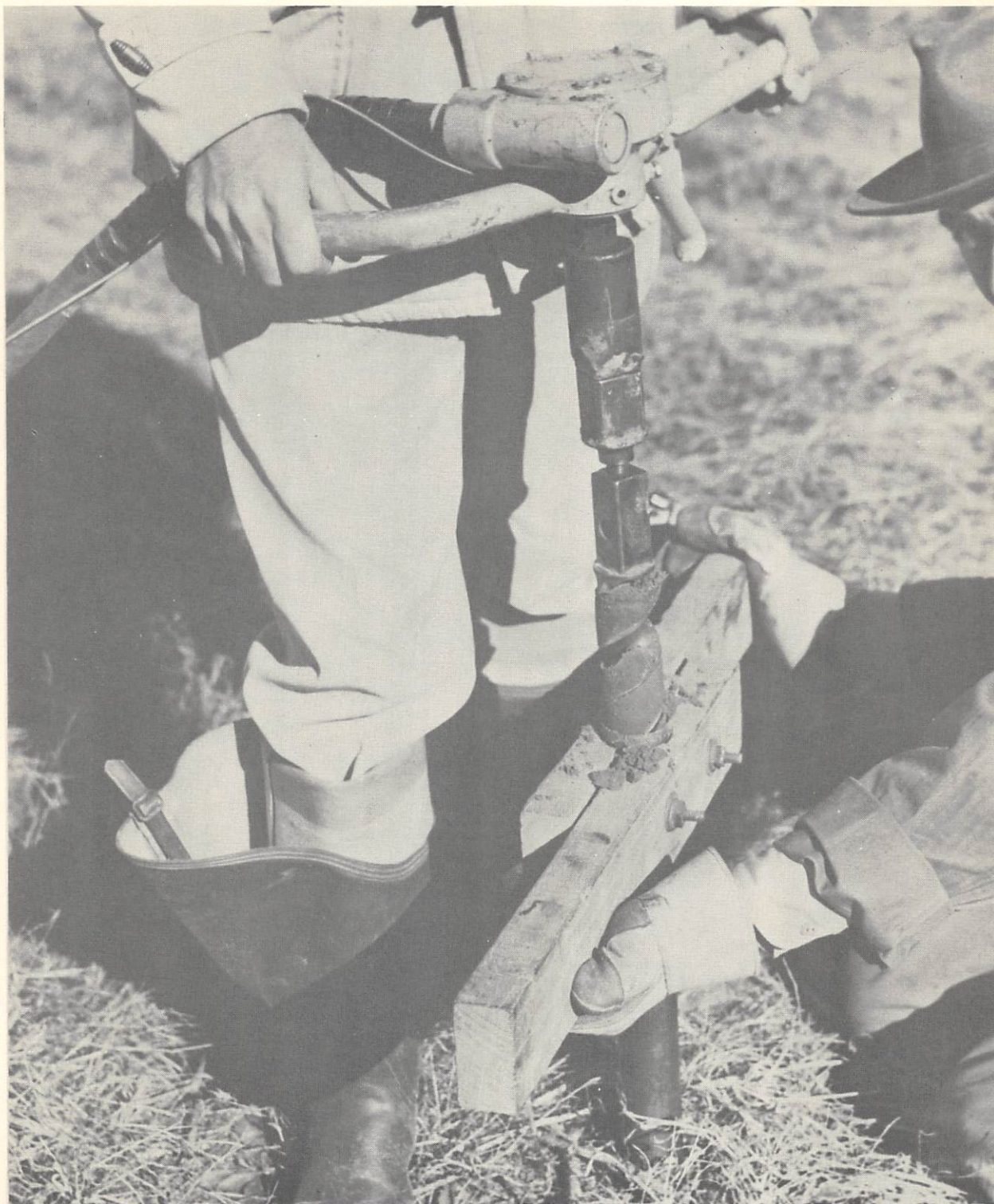
Fig. 5. Drilling operation showing assistant holding oak puller steady while driller operates power sampler.
