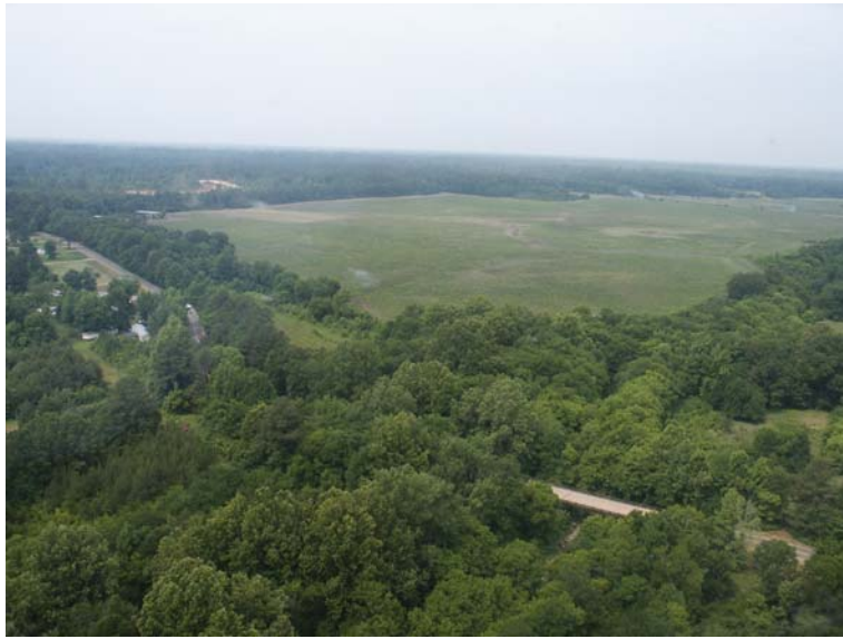
Figure 11 – View looking upstream from the junction of Darracott Road and James Creek located at the bridge in the lower right portion of the aerial photograph.
