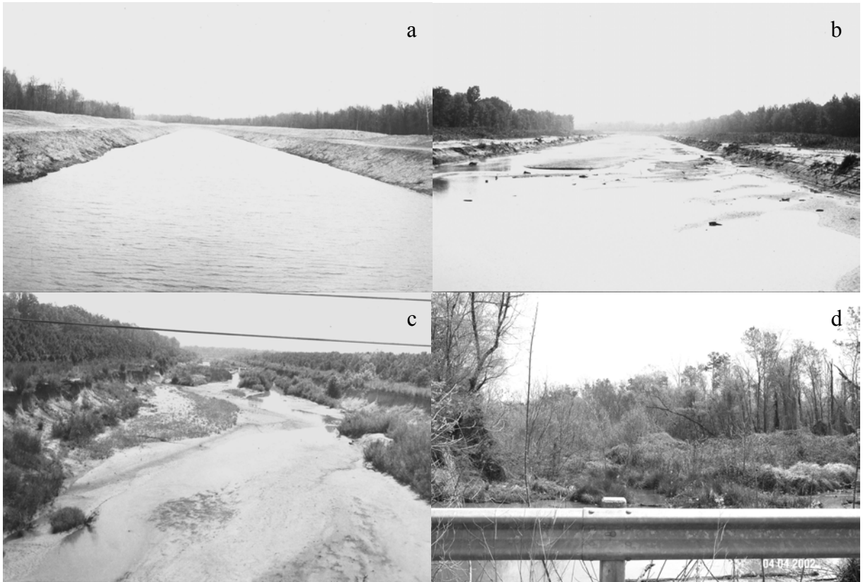
Figure 2 - Looking upstream from rkm 0 (the abandoned bridge just upstream of the downstream terminus of channelization works) in a.) November 1966; b.) May 1968; c.) September 1973; and d.) April 2002
