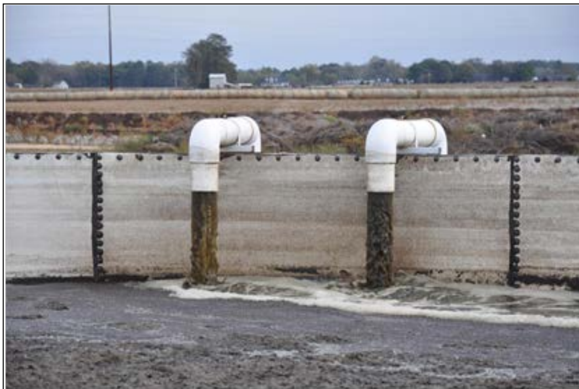
Raw manure from the finishing farm being transferred into the homogenization tank.
