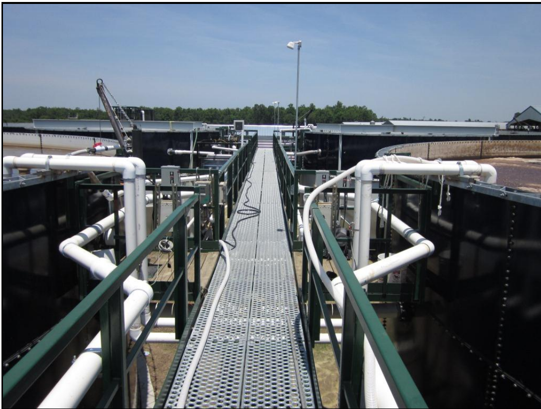
View of treatment plant from the catwalk.
