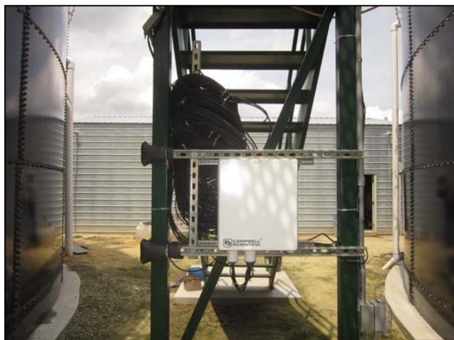
Picture at left shows box containing data-logger used to monitor plant liquid levels, temperatures, rain, pH and DO. Picture at right shows evaluation team member downloading data from a Doppler flow meter during weekly visits.
