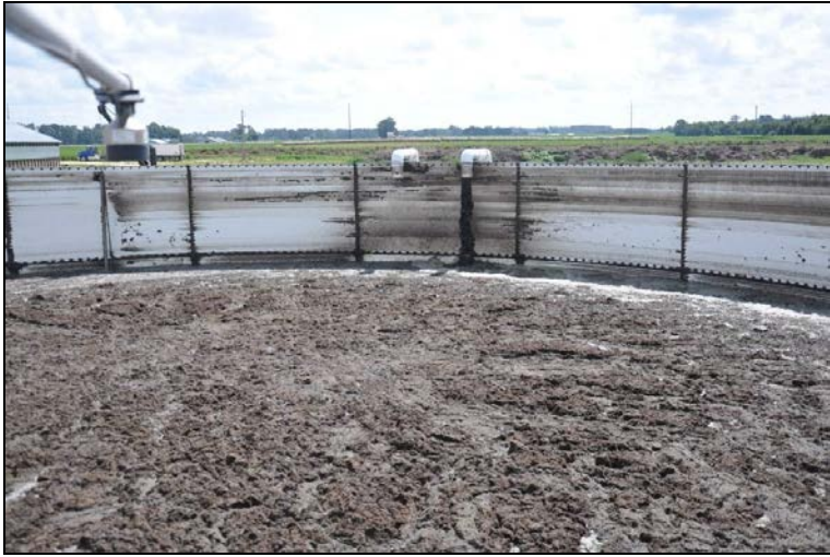
Homogenization tank receiving raw manure flush from finishers (left) and decanting tank sludge (right). In the upper left is the ultrasonic probe that monitored liquid levels.
