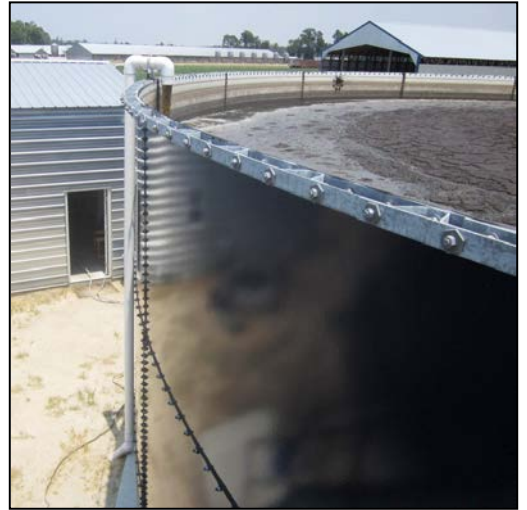
Homogenization tank receiving raw manure flush from finishers (left) and decanting tank sludge (right). In the upper left is the ultrasonic probe that monitored liquid levels.
