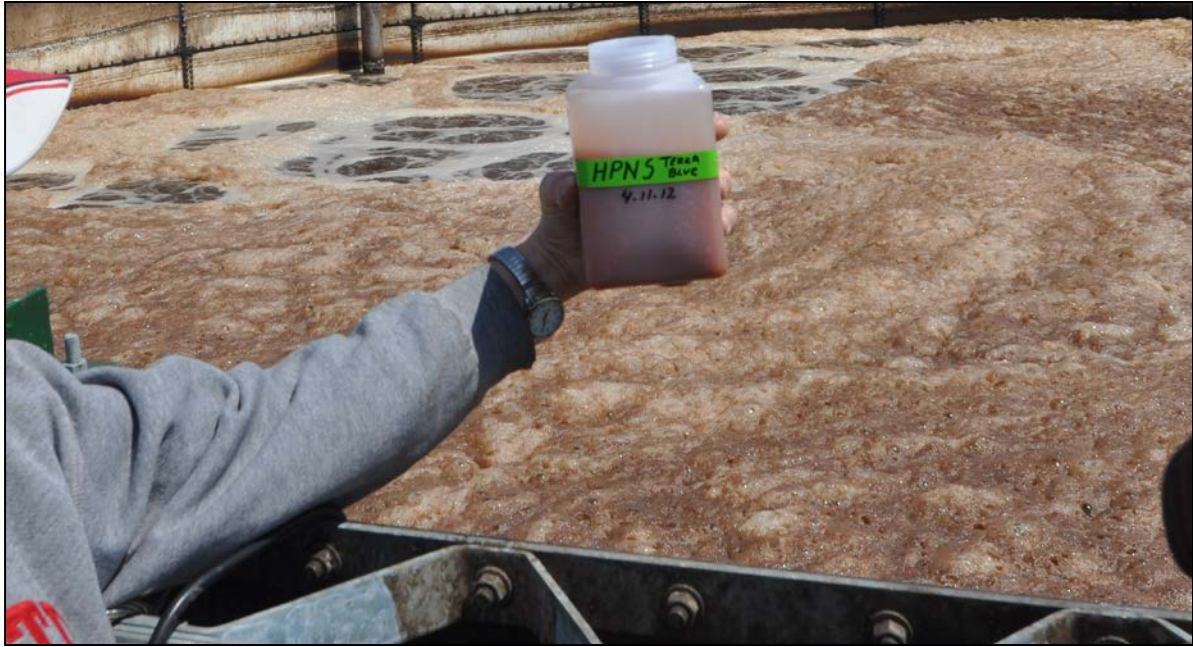
Start-up of the biological N removal unit with 1 liter of HPNS high performance nitrification sludge.
