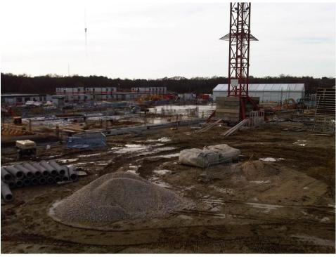
EARLY SITE WORKS: Drainage pits, ETP, concrete base slab
